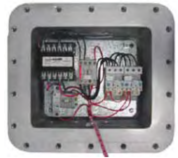
Typical Type 7/9 enclosure with large flange for oil and gas industry leaves little extra room for additional components.
