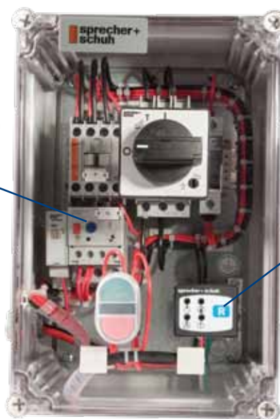
CEP7 Overload Relay and side module
